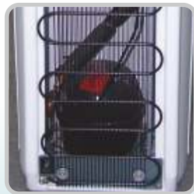
Hermetically sealed reciprocating compressor
