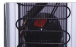
Hermetically sealed reciprocating Compressor
